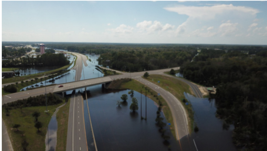
Flooding on I-95 in Robeson County after Hurricane Florence (2018)
